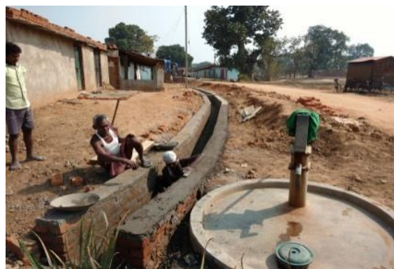
Drain Constructed under 14th FC
